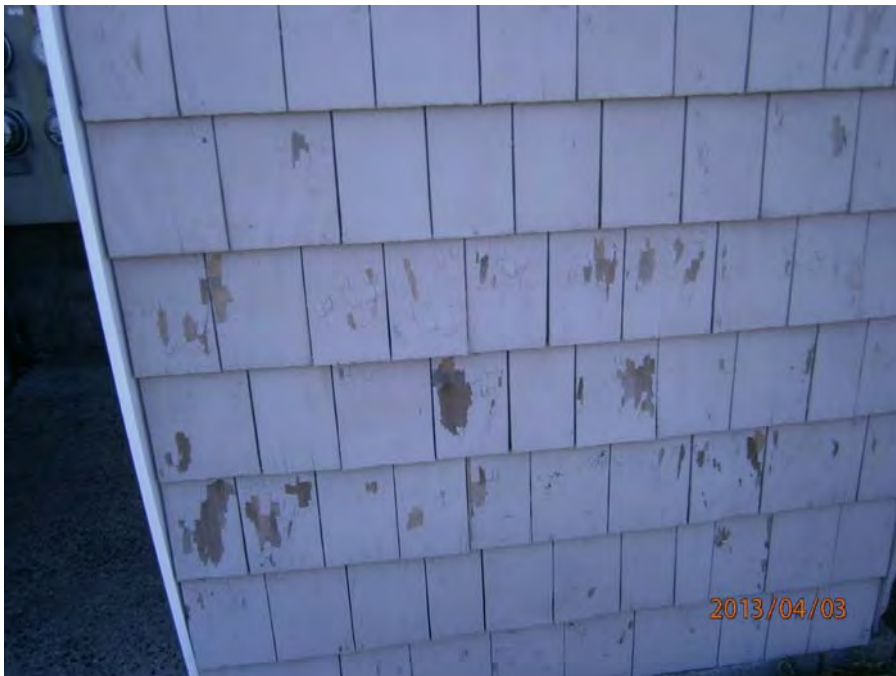
11. Wood siding paint peeling
