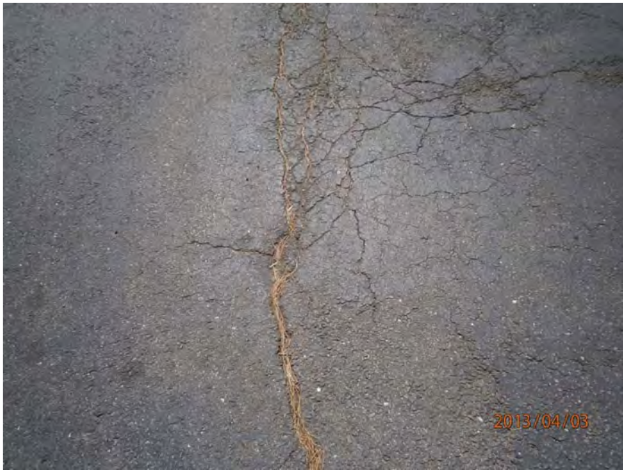
1. Asphalt exhibits cracks
