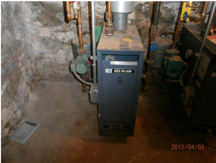
27. Typical unit boiler
