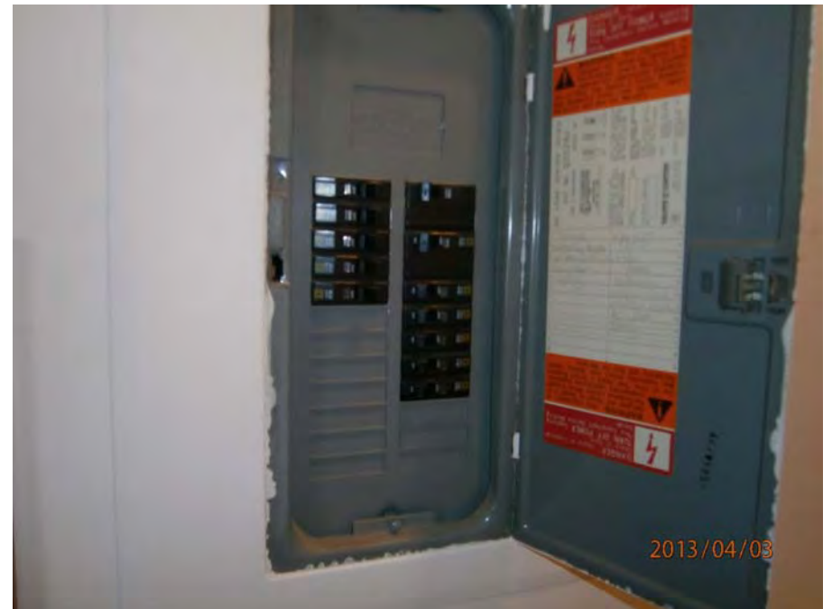
28. Unit circuit breaker panel
