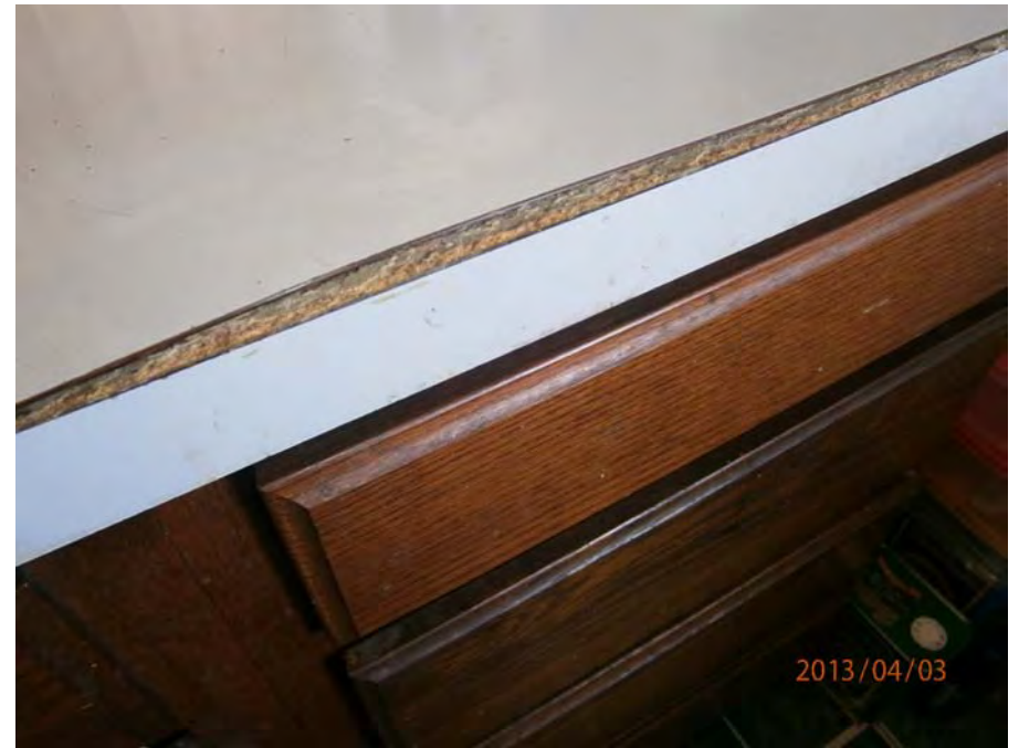
26. Unit countertop laminate damaged
