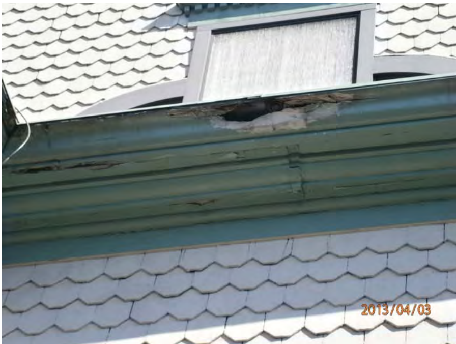
15. Box gutter damaged
